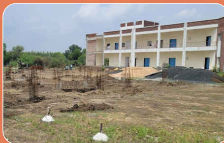
On going construction
